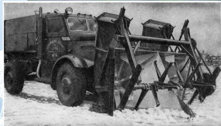
The rotating forks at the front end of this machine break down any kind of snow bank and feed it to blowers which throw it well off to one side
