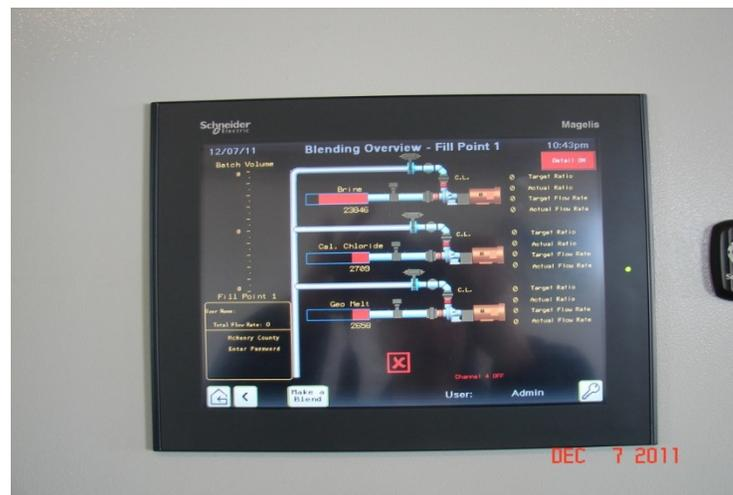
**This is the screen that shows the volume in storage, mixing ratios, volume pumped and all the other goodies**
