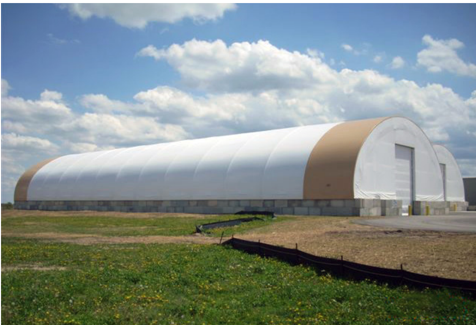
A shared facility in Des Moines, Iowa
